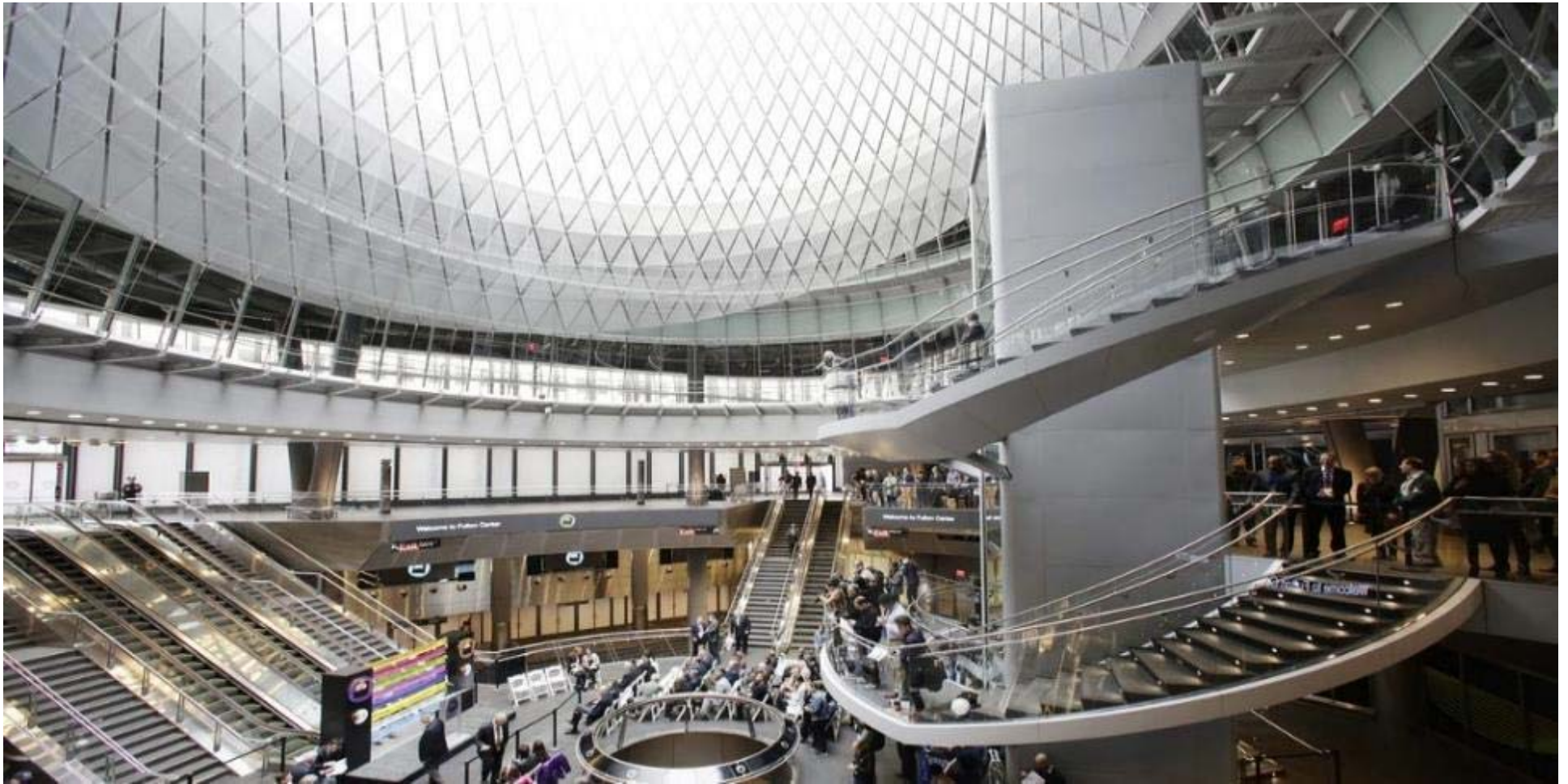
USA, New York. New York City Transit, NYCT. Fulton Station. MTA Arts and Design, Art in transit.
