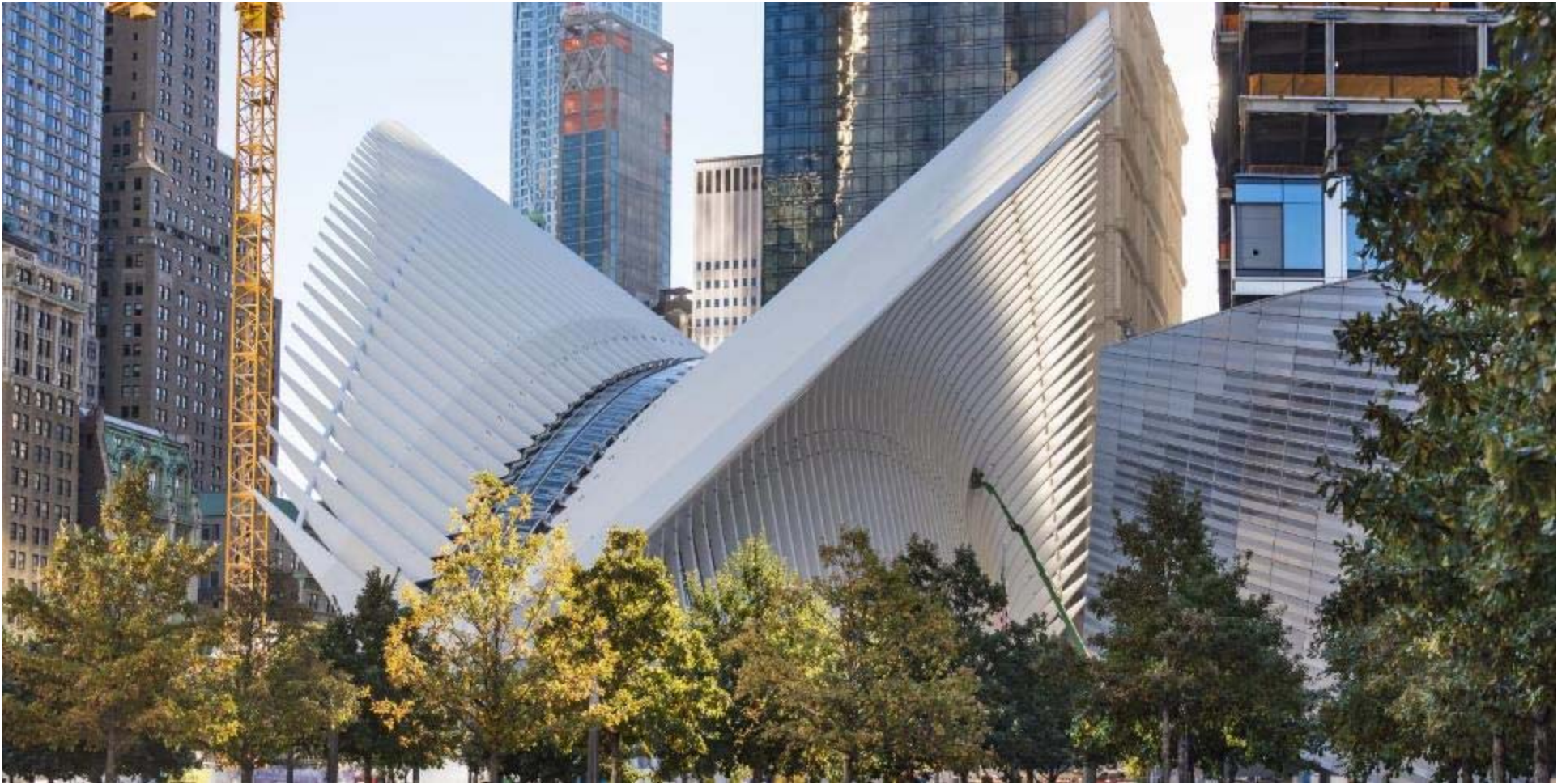
USA, New York. New York City Transit, NYCT. World Trade Center Station. Calatrava, architect.
